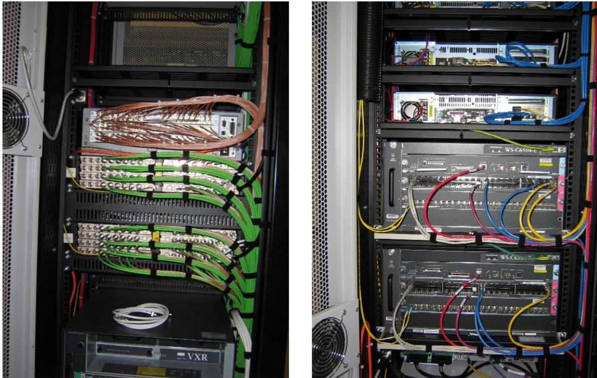
This is a typical Broadband Router set-up seen at the back, and the front. At the back, the Universal Broadband Router has a large number of TV equivalent channels that it connects to an analogue combining unit – this is all the green coaxial cable. At the front (shown on the right) these Broadband routers connect with the pair of local IP edge Routers (not shown), and an optical; fibre mesh of geographically diverse paths to the regional IP switches.
