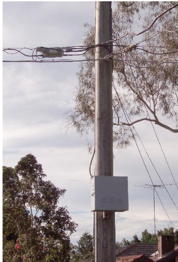
The coaxial cables are usually highly visible and usually sits about a metre below power lines suspended on poles.
