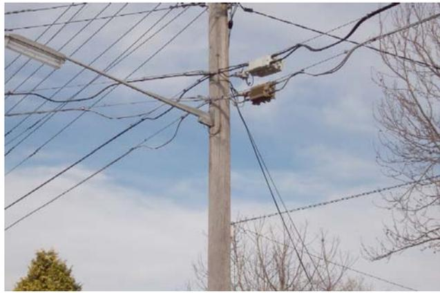
The prime reason that the coax cables are mounted on existing power poles is to minimise installation cost. It is far more expensive to bury coax cable and the associated amplifiers, splitters etc, so instead of following the standard in Australia of burying as much cabling as possible, competitive forces sought the cheap (and nasty) solution.
