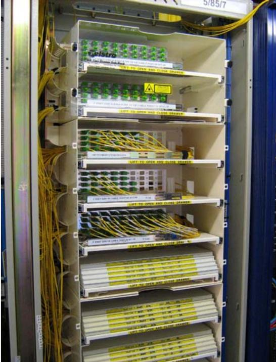
The Optical Patch Cords then connect into the Internet side of the DSLAM equipment shown here.
