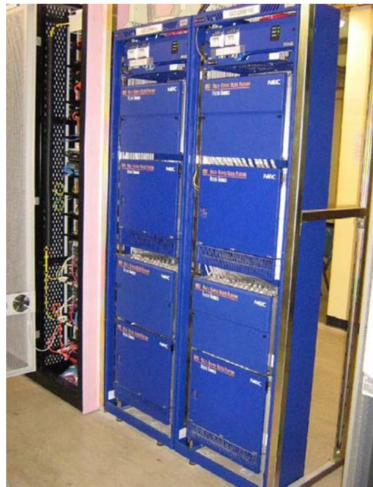
If the copper pairs have phone lines associated with them then the copper pairs come from the telephone switch to the Equipment side of the MDF, where they are then cross connected back to a cable on the Line side of the MDF that connects to the DSLAM filter Equipment side.
