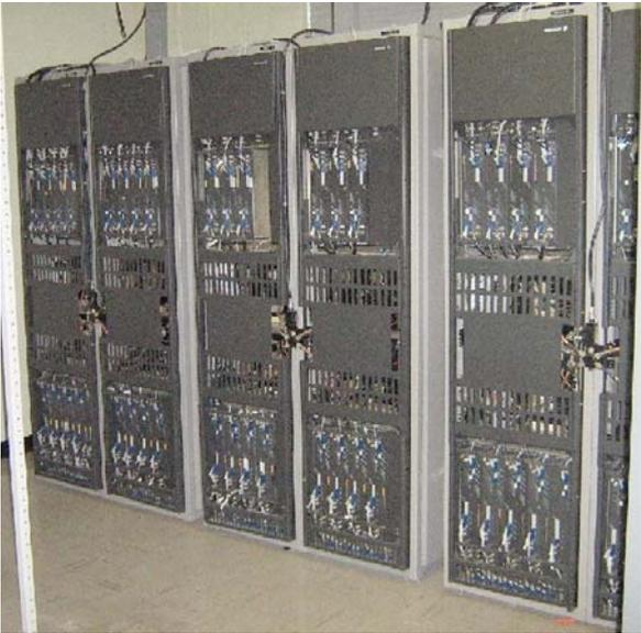
In this case the IEN / Backhaul interface point from the district switch in the same building is the DDF (shown on the left) in the Node (District) exchange with white sheathed coax cables feeding to the (co-located in this case) radio base station transceivers, (shown on the right hand picture).
