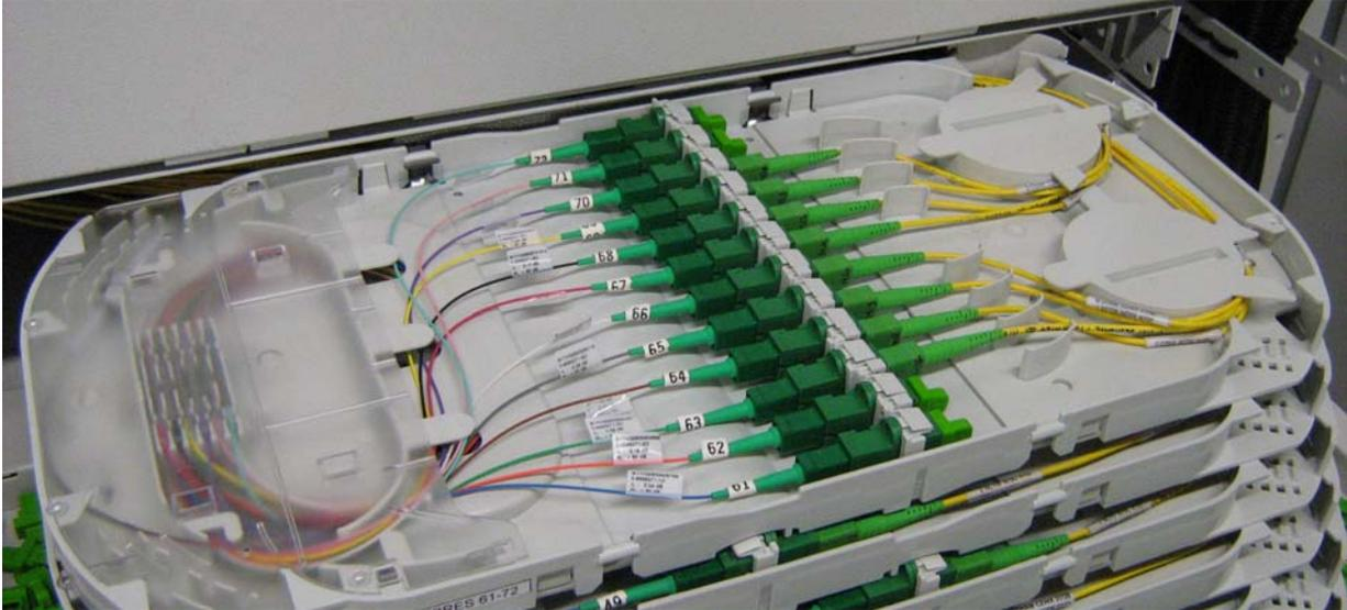
The picture above is an Optical Distribution Frame (ODF), where the optical patch leads on the right hand side connect to an optical cable on the left hand side through optical splices held in the far left plastic ribs. This optical cable would then be run underground to the distant site (as far as 90 km away) and then connect with the radio base station equipment like the mini-transceivers shown in the picture below.
