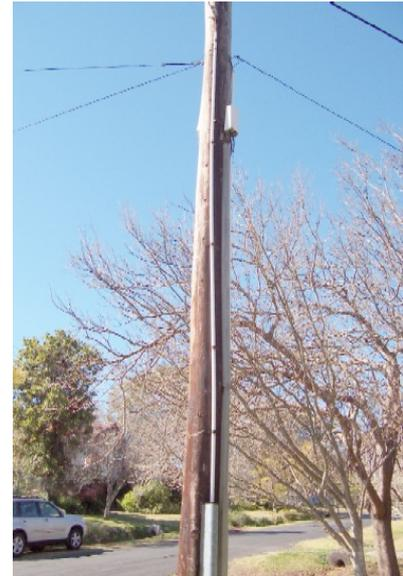
This is a typical arrangement with an aerial lead-in from a telephone pole. Note that there is a single cable that runs up the pole on the right hand side (on the shady side) inside a wooden protective cover.
