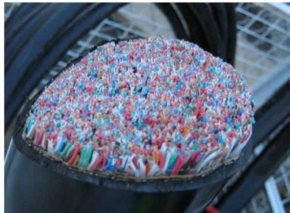
From about the early 1980's most cable supplied is polyethylene insulated included a petroleum Gel to keep the water away from where air would be between insulated pairs.
