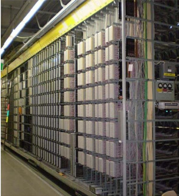
In most cases where there is Pair Gain equipment including Digital Services Line Access Multiplexer (DSLAM) equipment for asymmetrical (data transfer speed) Digital Services Line (ADSL). It is common to terminate one side of this equipment as though it was main cable (on the Drop side of the MDF).
