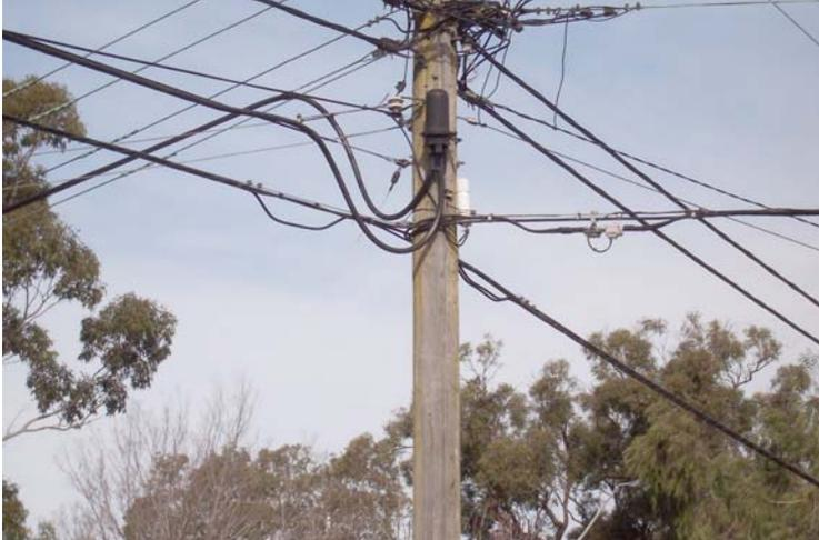
This is a fairly large Aerial Cable coming across a major road (from the left hand side of the picture), where it is anchored with a wire rope. The Cable then loops down then up into a black canister where it is joined into another cable and strung under the power lines alongside the major road.
