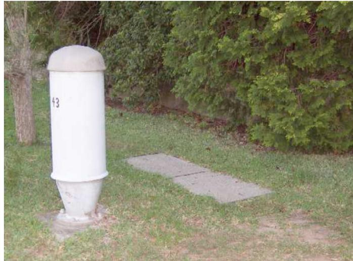
The picture above right shows a pillar in the foreground, used to join a main cable from the local exchange to several minor cables.
