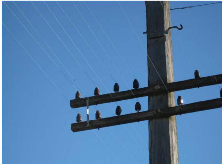
Because the wire diameter was relatively large in comparison to the now standard 0.40 mm as used in urban pair cable technology, the series resistance component was rather low, so the characteristic impedance usually settled on near to 600 ohms. This should explain why so much early telecomms equipment and virtually all audio / studio equipment were based on “600 ohms” as the “standard impedance”.
