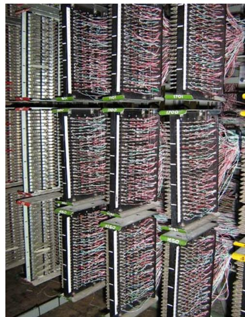
These MDF Terminating blocks would have been used for terminating open / aerial wires (like seen in some country areas and sometimes still remaining beside some rail lines. Underground cable is far less prone to damage by induced lightning but in
