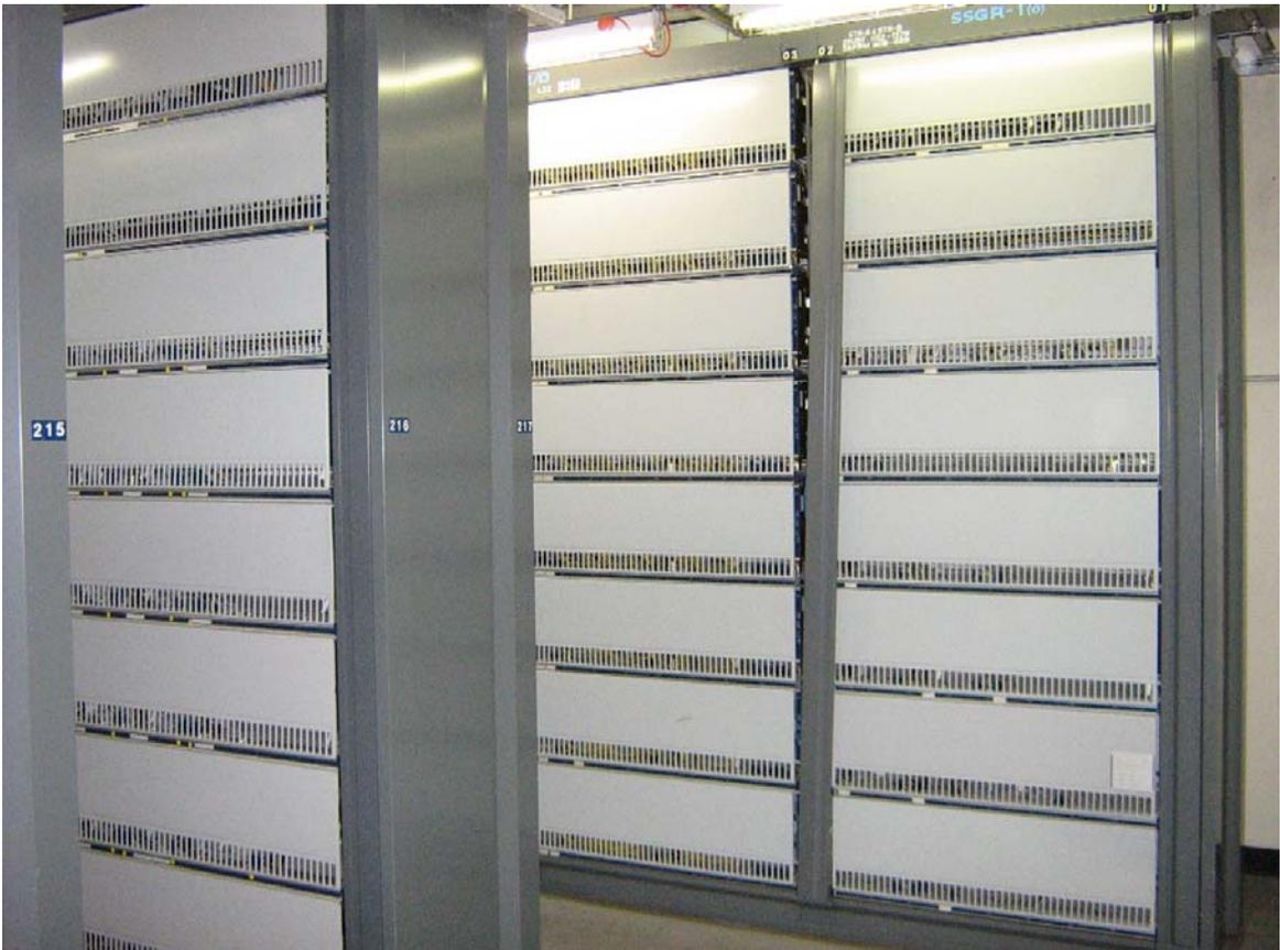
The first version emulated the Crossbar processors with a dual computer, but used reed relays for subscriber switching and included common analogue to digital stream G.703 conversions. These switches had maintenance requirements that were 10 to 500 times less than Crossbar switches, making digital switching very cost-effective.
