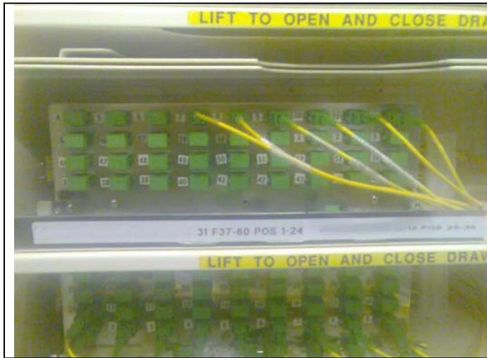
This is a close-up of a typical OF Patch Panel shelf showing the individual (Green) connectors for each fibre in a cable. The (Yellow) Patch Cable is quite thick (about 2 to 3 mm in diameter) to protect the 'hair thickness' fibre strand.
