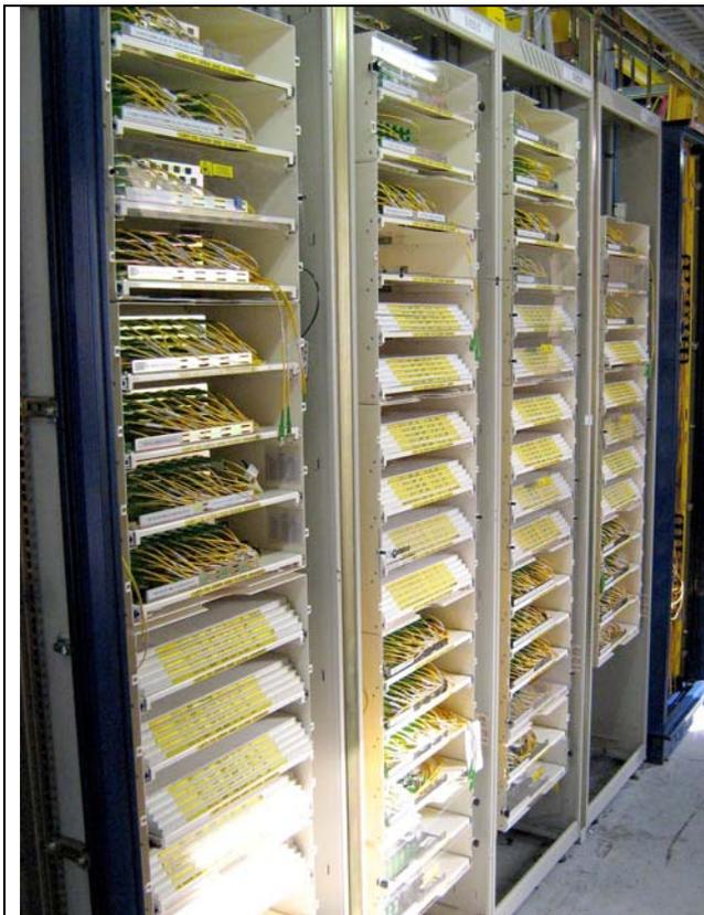
Here is a suite of racks containing Optical Fibre trays and Terminating Patch Panels, where Optical Fibre (OF) cables fibres are terminated to the patch panels. Most OF cables used for Backhaul Network purposes carry 120, 240 or 312 fibres per cable.
