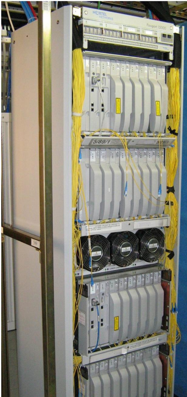
The in non-metropolitan areas the transmission system would be a series of intersecting physical SDH rings that would connect to another two or three other District / Node exchange switches like this one, and the Dual Parent Regional or Main / Primary Router / Switches would connect to these Local exchange Router / Switches to form a 'Double Centred Star' Network - for reliability, redundancy and high data throughput.
